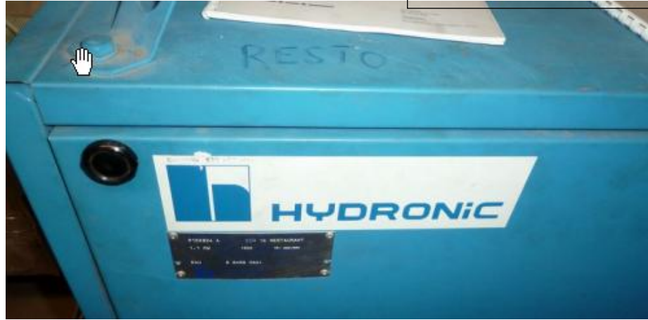
CTA Resto – 1500m 3 /h Hydronic CCH 16
